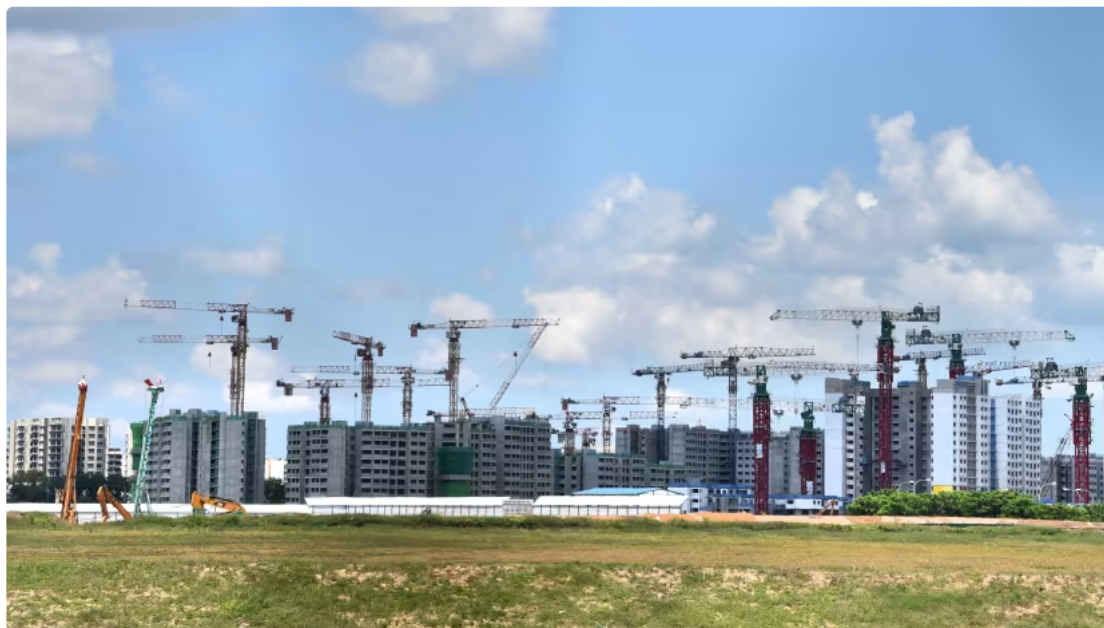
HDB BTO flats in Tampines under construction. (File photo: Jeremy Long)
